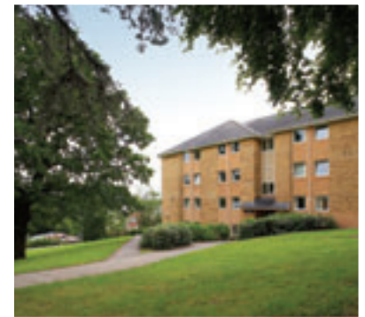
Above: Plas Gwyn Halls of Residence.
